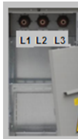
Figure 42– Marking of the phases
