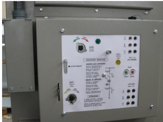
Figure 40 – Measurement Functional Unit Front Panel Example
