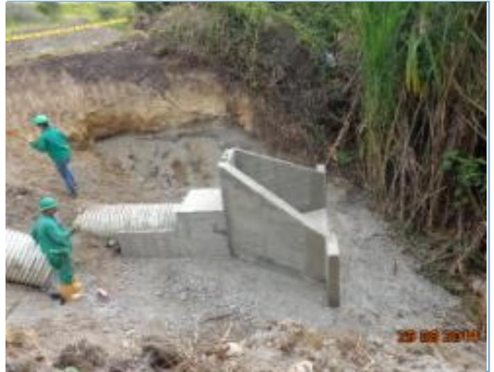
Foto 1. Tanque Septico PTAR.
