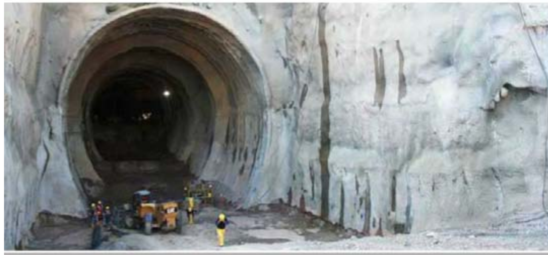
Deviation Tunnel Entrance
