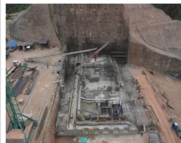
Works at the spillway Control Structure
