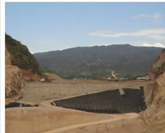
Stage 1 dam fill material
