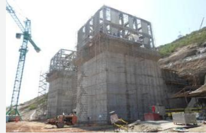
Inlet: Assembly of wicker structure
