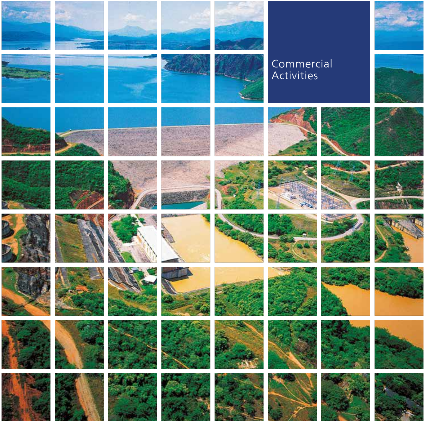
Betania Hydroelectric Plant, Huila
