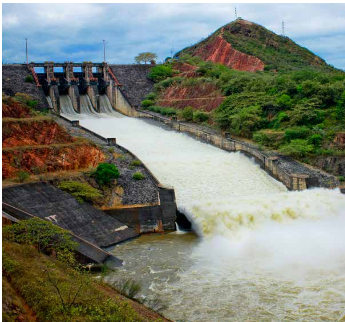
Betania hydroelectric station
