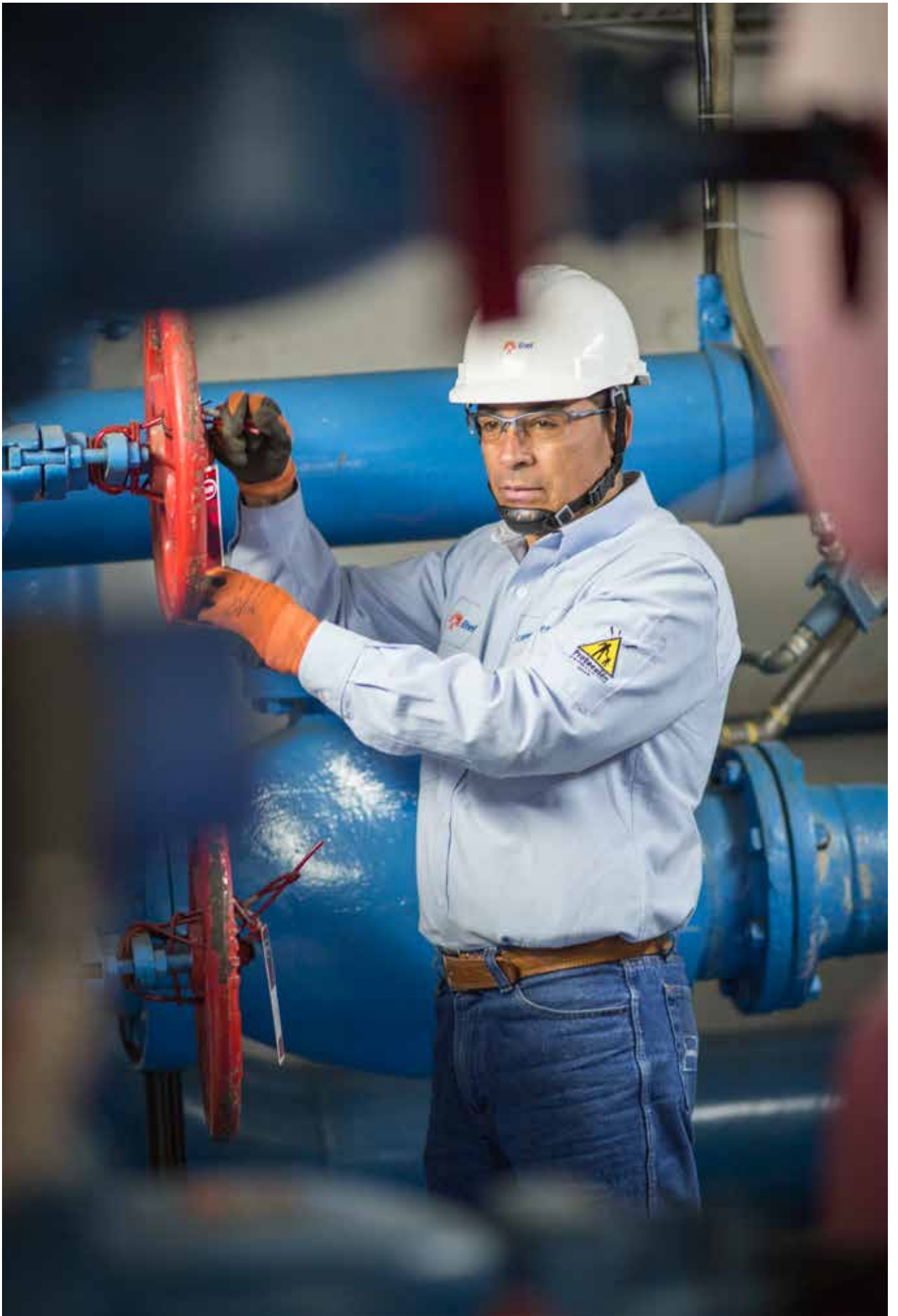
Charquito Hydroelectric station
