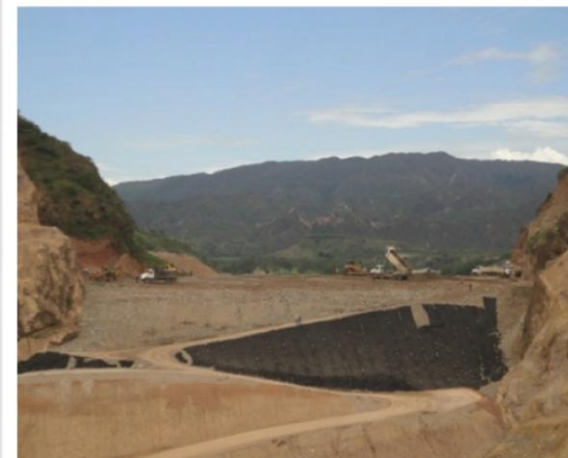
Stage 1 dam fill material
