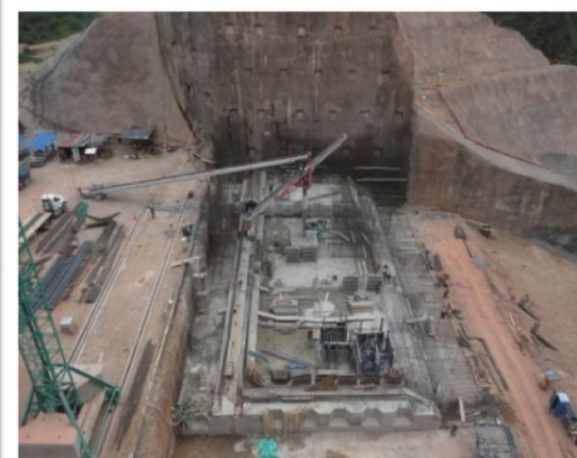
Works at the spillway Control Structure
