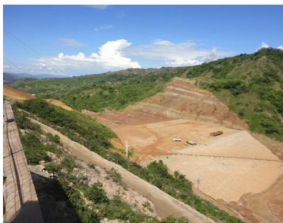
No. 1 Gate well Excavation
