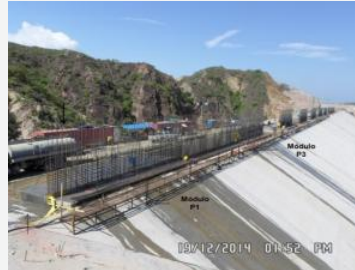
Damn – Reinforcing steel Parapeto wall
